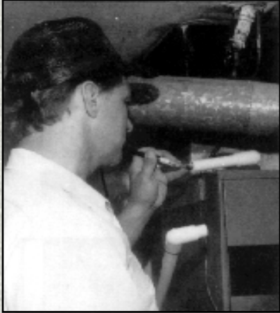
The drain pipe was cut to sniff the evap section.
